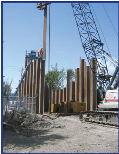
Build, Inc. driving sheet pile (Photo by Jasen Bennie)
