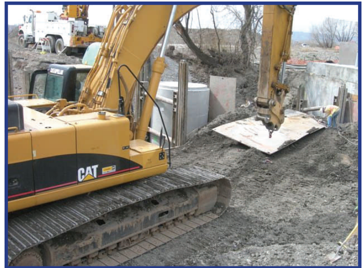
345 excavator installing trench plate for earth retention (Photo by Jasen Bennie)
