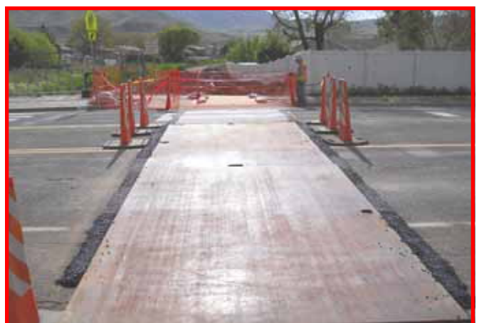
Trench plate over canal to allow uninterrupted traffic flow.
