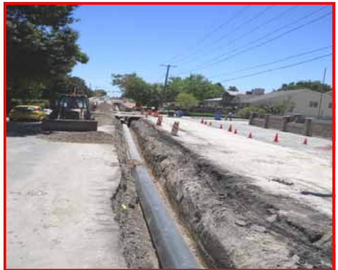
Preparing to backfill a 1200 LF stretch of pipe.
