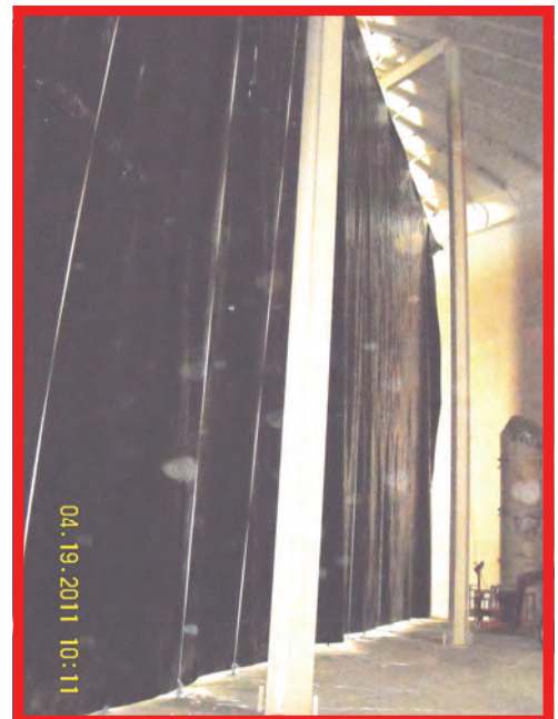
Hoisting baffles into place. Photo by Joe Allen
