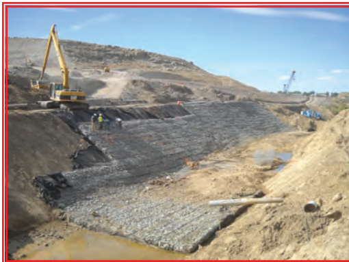
Gabion installation.
