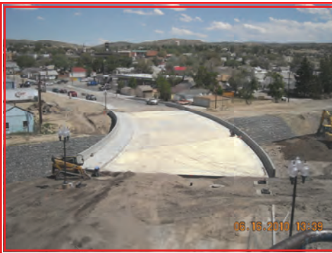
Barrier rebar installation.
