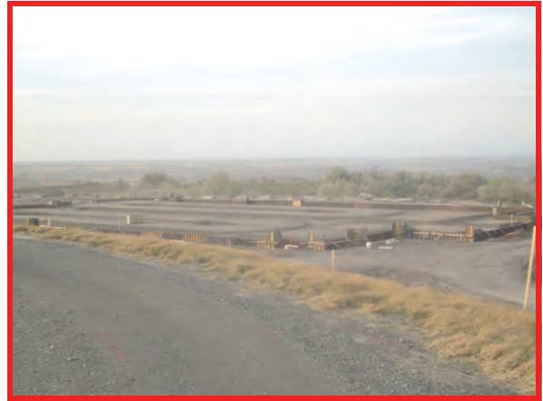
Oxidation ditch slab edge forms.
