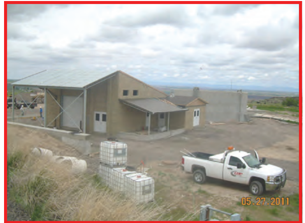
Completed bio-solids building, foreground; completed bio-solids tank, background.
