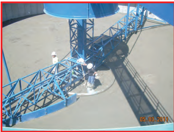
Grouting interior slab of clarifier tank.
