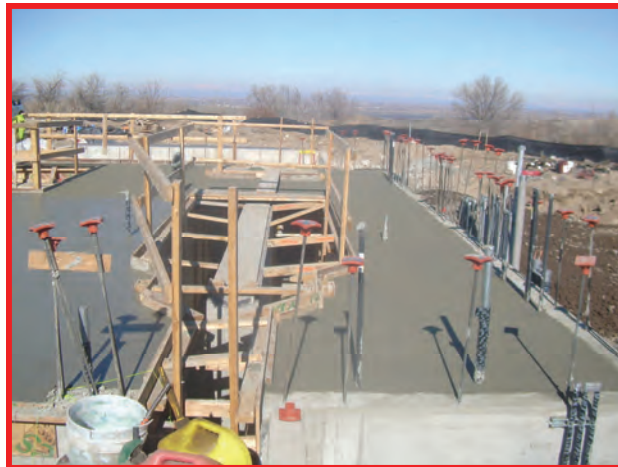
Headworks building floor slab.
