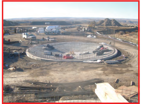
Slab and wall rebar for bio-solids tank.
