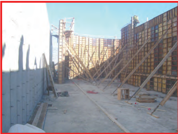
Interior of oxidation ditch.
