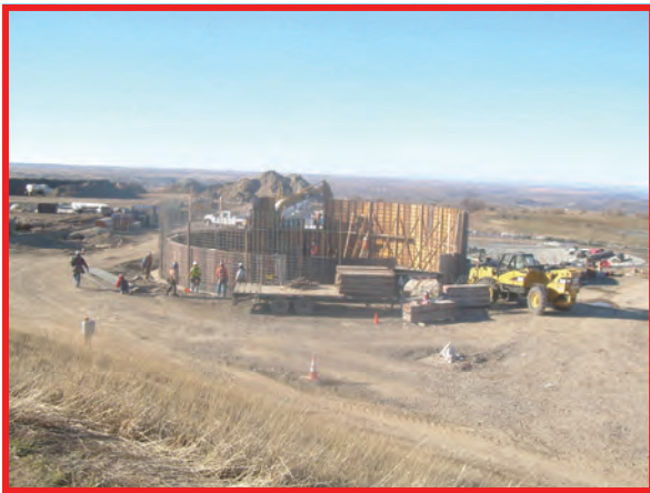
Bio-solids tank wall forms.
