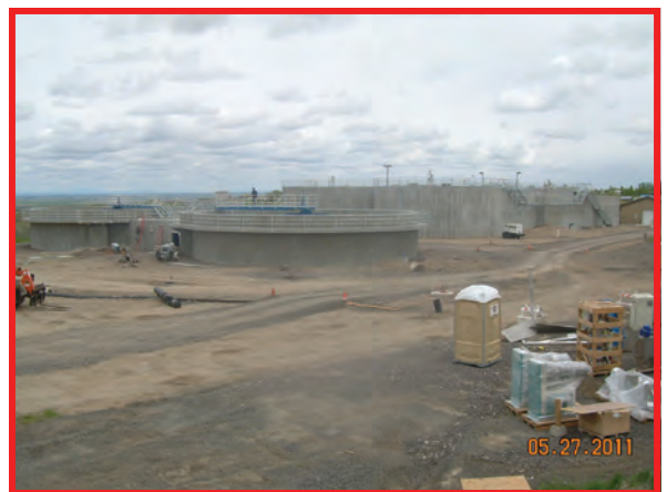
Completed clarifiers & RAS/WAS, foreground; completed oxidation ditch, background.
