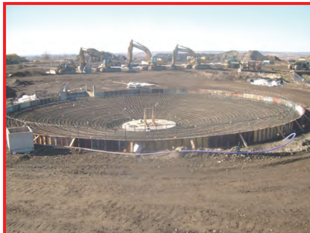
Bio-solids tank slab forms and rebar.
