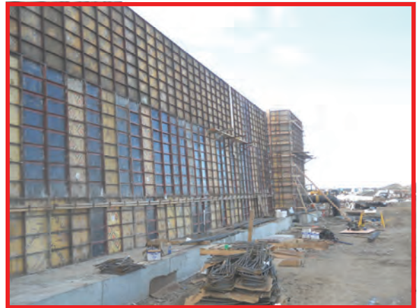
Exterior wall of oxidation ditch.
