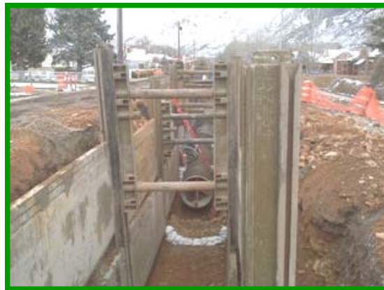
Slide rail shoring system.
