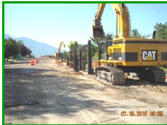
Toby McFarlane's crew with shoring system stair-stepping downhill.
