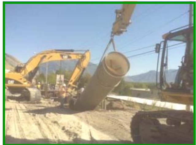
CAT 365 and 345 excavators setting a pipe. Photo by Doug Teller
