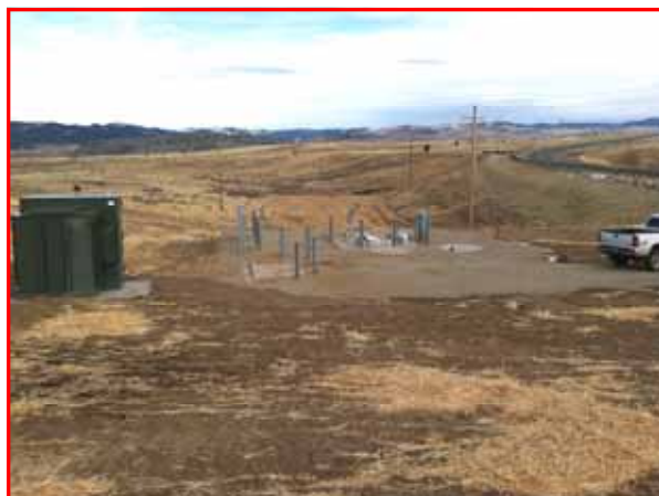
Completed Lift Station #1.
