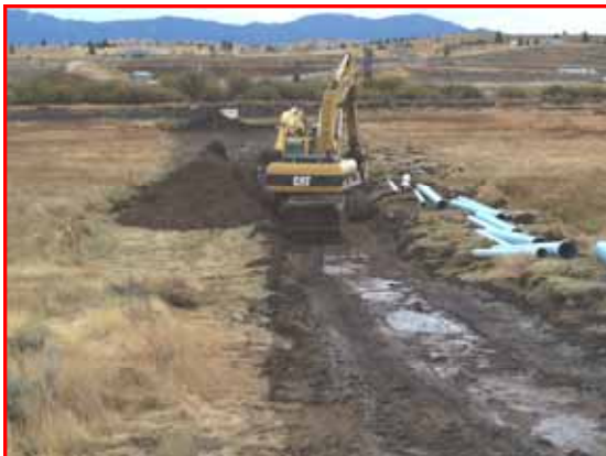
Crew #1 laying triple-barrel force main through wetlands. Photo by Doug Teller
