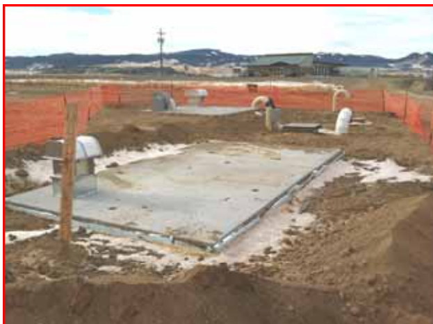
Lift Station #2 completed to surface. Photo by Doug Teller
