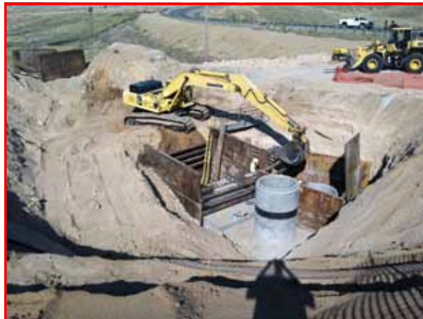
Deep foundations and lower structures at Lift Station #1.
