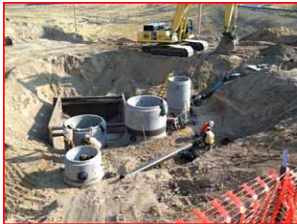
Lift Station #1 structures and interconnecting yard piping.
