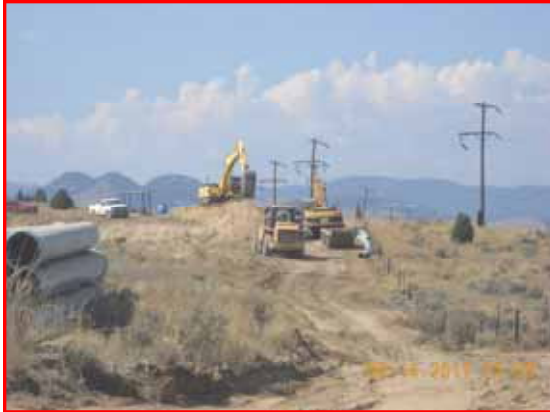
Crew #1 in overland portion of 14" force main. Photo by Greg Schied
