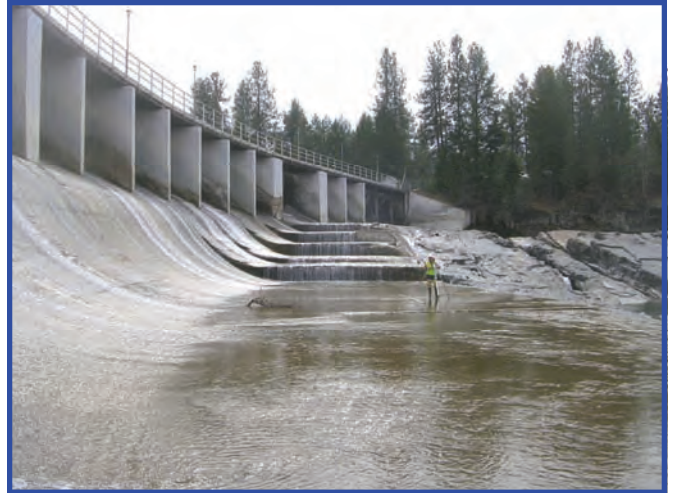
Apron height change of 24 feet following curve of dam.
