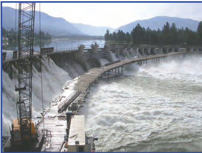
Access bridge during heavy spring runoff.
