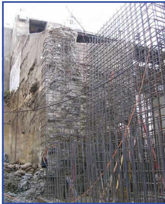
Connecting the fish ladder to the existing log sluice structure.
