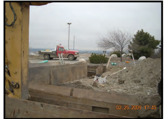
Above and below: Deep sewer installation with challenging existing utilities.
