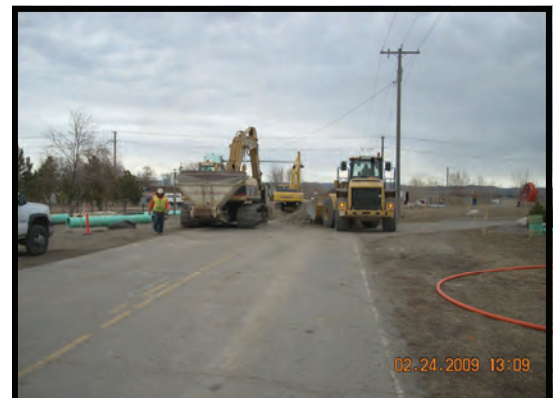
Above and below: Deep sewer installation with challenging existing utilities.
