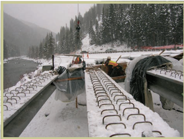
Decking being built—Swan Creek
