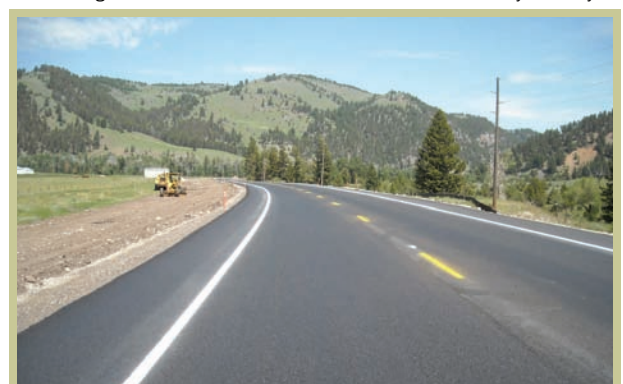
Finishing up Hwy 191 improvements near Big Sky
