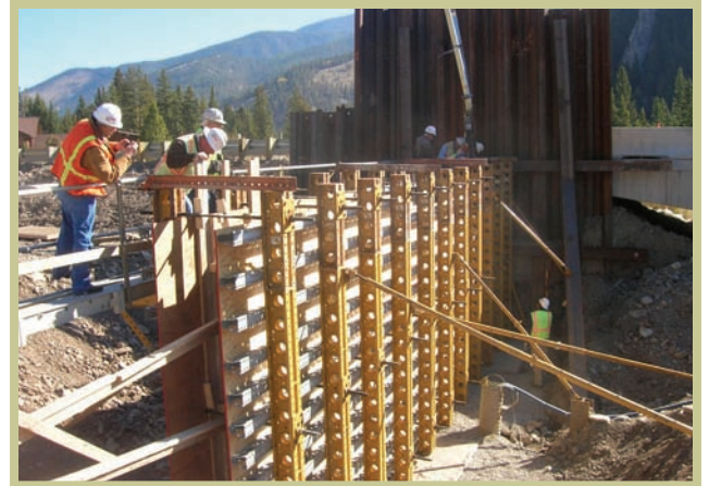
Crew building bridge forms—W. Fork Gallatin River Photo by George Werhonig
