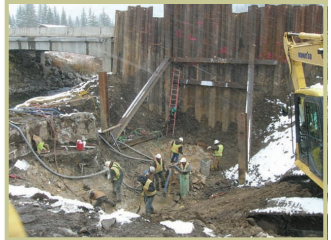
Cofferdam—W. Fork Gallatin River
