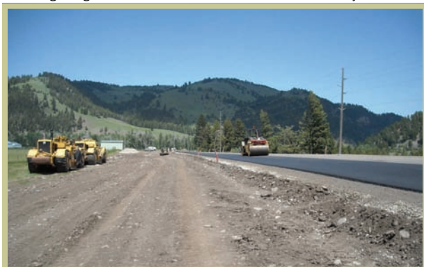
Road work along Hwy 191 near Big Sky
