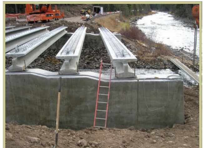
Bridge beams—Swan Creek
